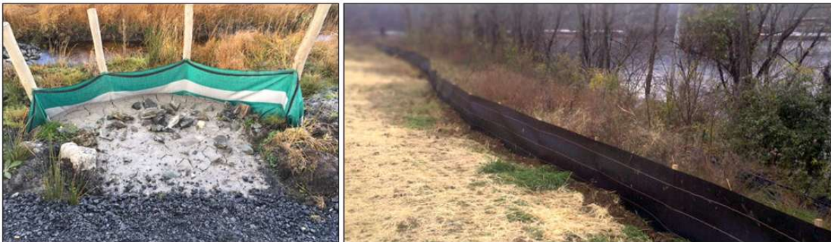
Figure 5-2: Silt fencing measures (Source: Hy-Tex (UK) Ltd. (left) and Thrace Group (right))
