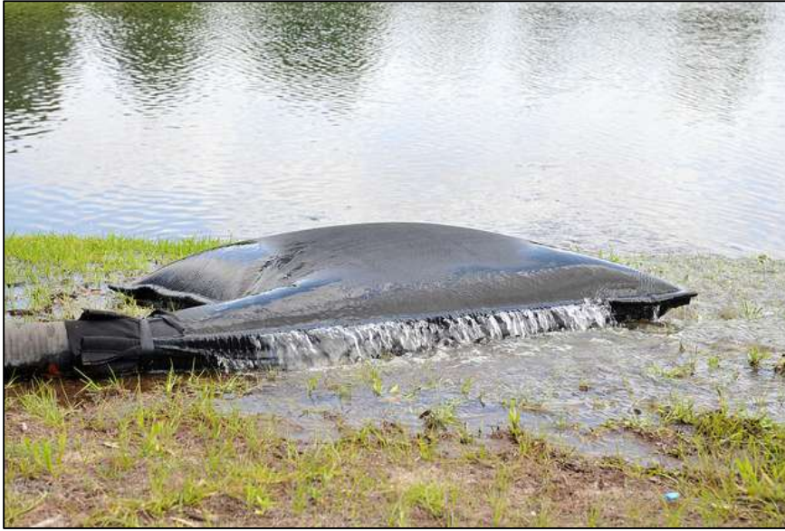
Figure 5-3: Silt/Dewatering bag (Source: Hy-Tex (UK) Ltd.)
